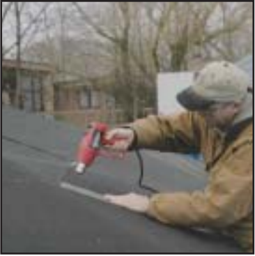
Weld Roofing Felt
