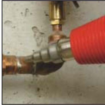
Solder Copper Pipe
